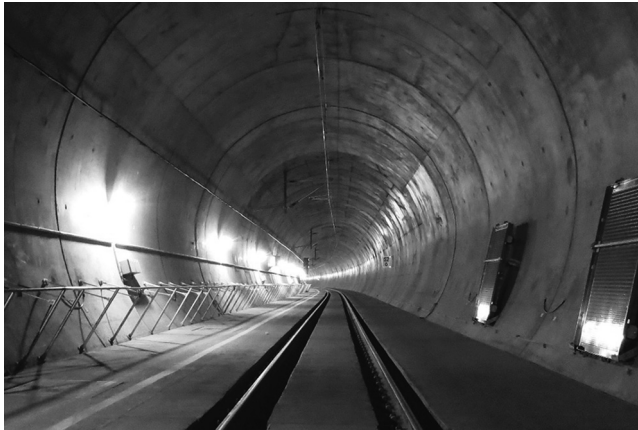
Fig. 1.8 NBU system in the New Kaiser Wilhelm Tunnel (source: Bilfinger)
