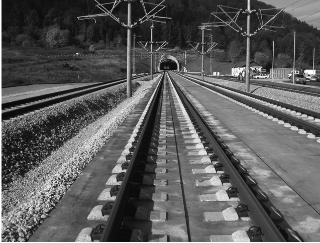
Fig. 1.9 Rheda 2000 system (source: Institute of Road, Railway & Airfield Construction, Munich TU)
