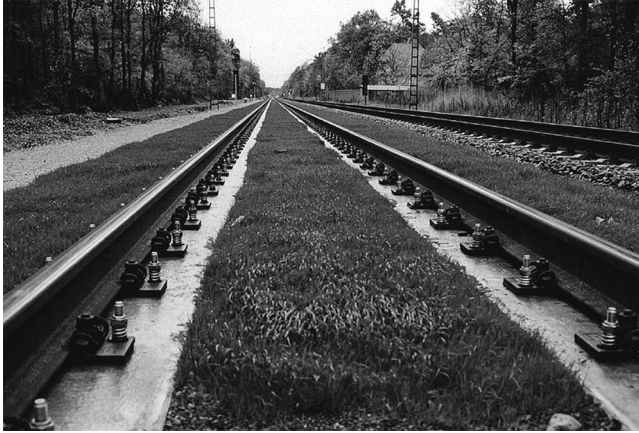
Fig. 1.6 Ballastless track with intermediate grass strip at Waghäusel near Karlsruhe (source: Institute of Road, Railway & Airfield Construction, Munich TU)
