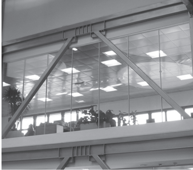
Figure 1.3 Valorization of internal braces (InterPuls, Reggio Emilia, Italy).
