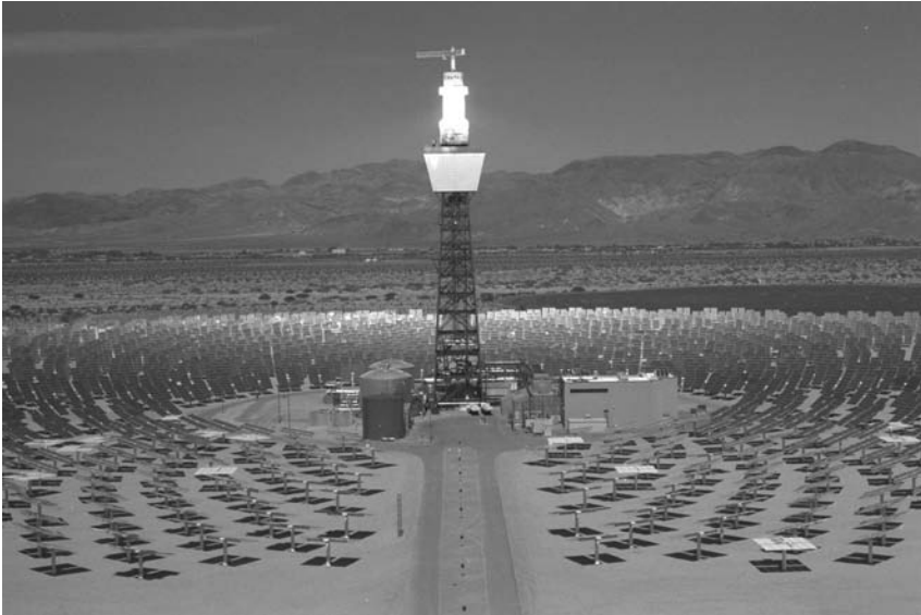
Figure 2.1 The solar tower power plant Solar TWO (Barstow, California) (SANDIA).
