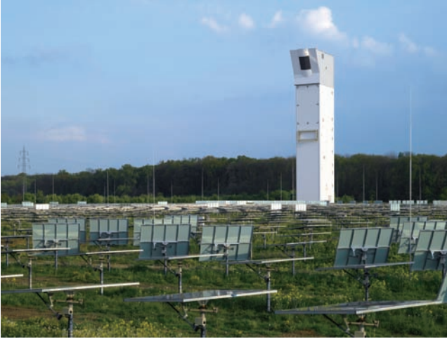
Figure 2.13 Heliostats similar to those in Figure 2.12, here in the solar test field at Jülich, Germany (Photo Kraftanlagen München).
