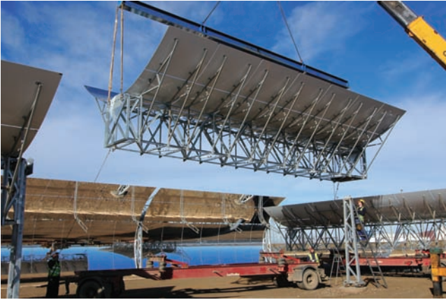
Figure 2.17 Mounting of a parabolic trough collector in the field (SBP).
