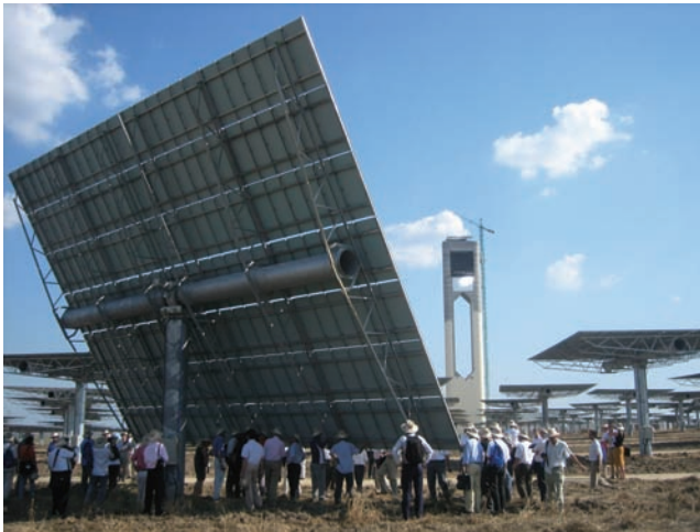
Figure 2.5 The solar tower power plant PS 10 near Seville (Spain): 624 Heliostats (121 m 2 ) (Photo: DLR).
