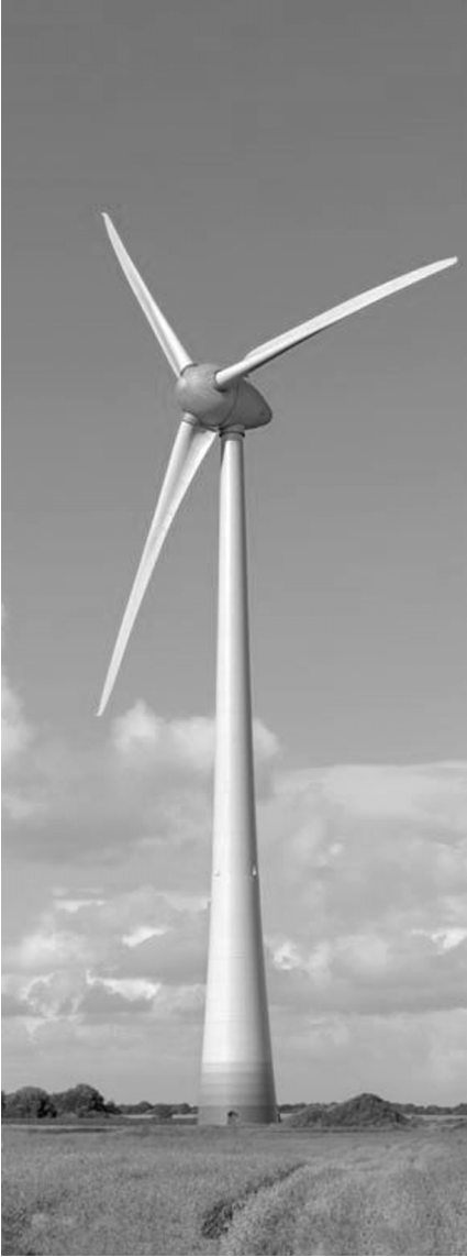
Figure 1.9 Enercon model E-126 7.5 MW wind turbine. The hub height is 135 m. The specifications say that the machine can be set to cut off at a chosen wind speed in the range 28–34 m/s. From the text one would extrapolate
