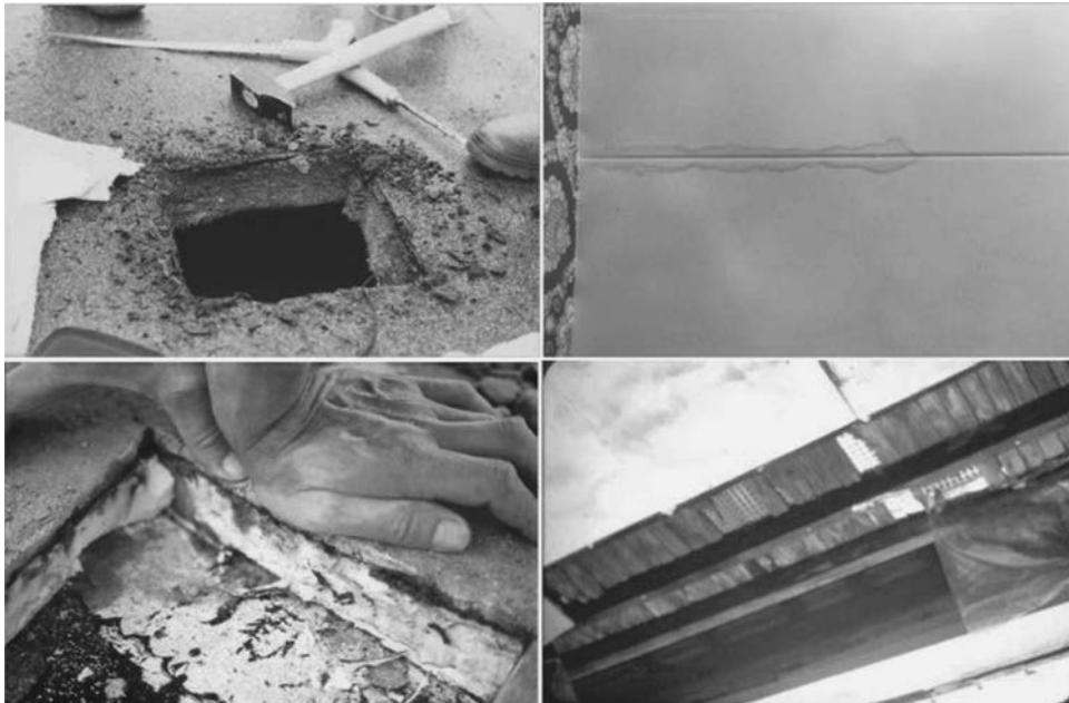
Figure 4.25 Damage caused by interstitial condensation.
