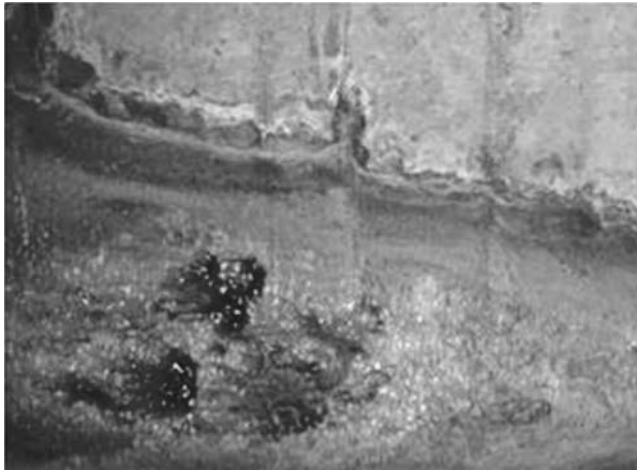
Figure 4.19 Natatorium, leaking swimming pool wall.
