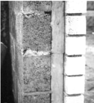
Fig. 1.4 Filled cavity wall
