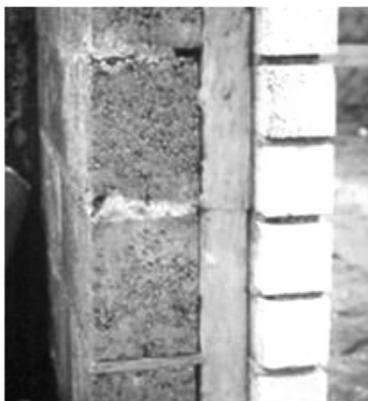
**Fig. 1.4** Filled cavity wall
