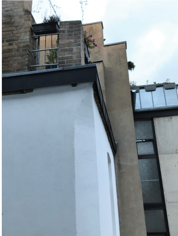
Figure 1.5 Wall from outside (private photo).
