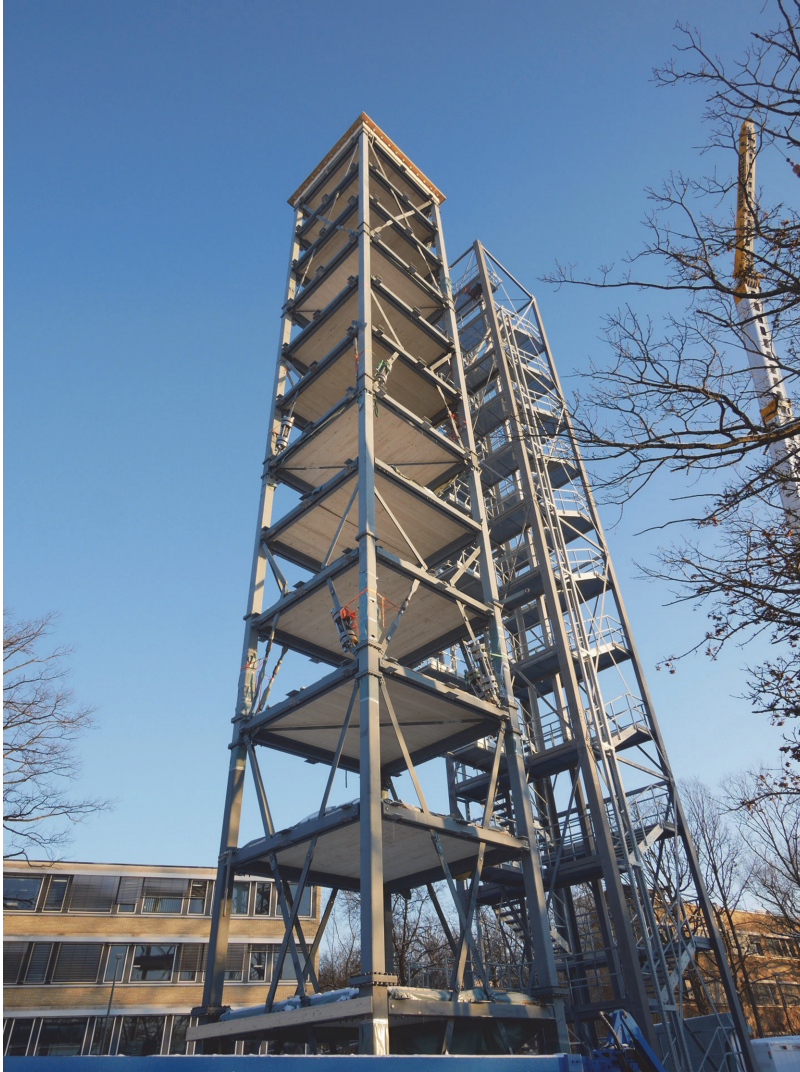
Figure 3-1 Demonstrator high-rise with integrated adaptive elements. (© Weidner ILEK)
