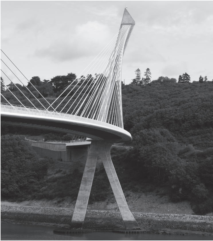
Figure 1.1 Concrete shaped to the flow of forces: pylon of the Pont de Terenez (France). Picture: Thomas Putke-Hohmann.
