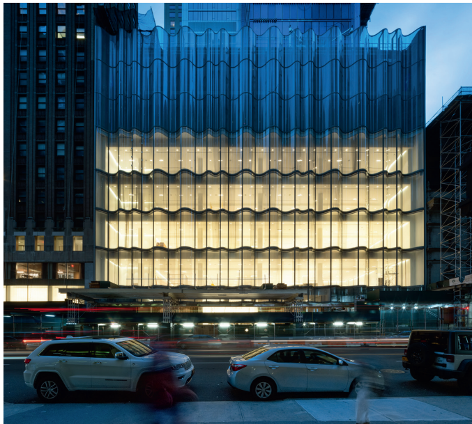
Bild 10 Fassade des Nordstrom Flagship Store in New York City (© Nic Lehoux architectural photography)
