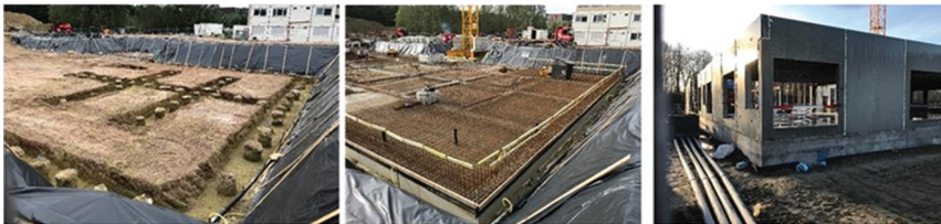
The contractor builds
