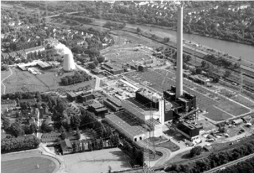
Figure 1.4 Municipal waste incineration power plant with flue gas cleaning and waste water treatment for RWE Power AG in Essen-Karnap. The plant has a capacity of approx. 750 000 t/a. The total investment amounted to approx. 500 m €.
