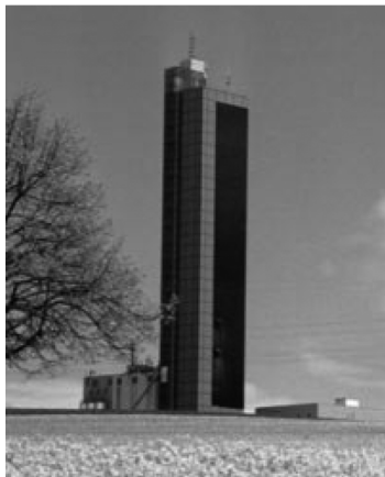
Figure 1.21 (a) The façade of Ulm's wheat silo that consists of 1300 CIS photovoltaic modules with a total output of 98 kWp (Photo courtesy: Solarserver.de). (b) The solar wall of 640 m 2 at Berlin's Braun Institute. (Photo courtesy: Forschungsverbund Berlin).
