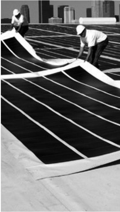
Figure 1.33 Easy installation by Solar Integrated of a lightweight white single-ply roofing membrane, and thin-film photovoltaic membrane transforms commercial and industrial roofs in clean energy generators. (Source. Solar Integrated).
