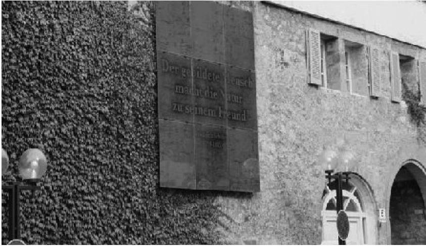
Figure 1.26 Semitransparent CIS solar panels coating the entrance of Schiller's home in Marbach am Neckar. (Photo courtesy: EU Commission).
