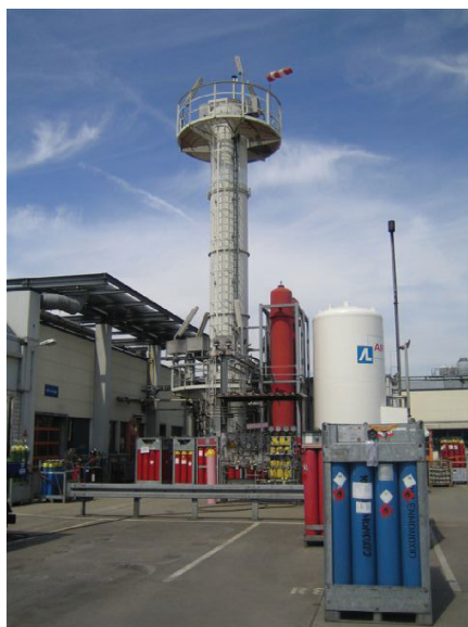
Figure 1.11 Separation column for the purification of carbon monoxide [24].
