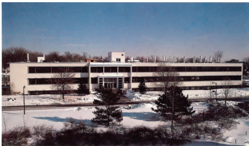
Figure 1.1 National Research Council of Canada Building M-12 on the NRC Montreal Road campus in Ottawa, home of the Colloid Chemistry (later Colloid and Clathrate Chemistry) group until 1990. Source: Reproduced with permission from the National Research Council.
