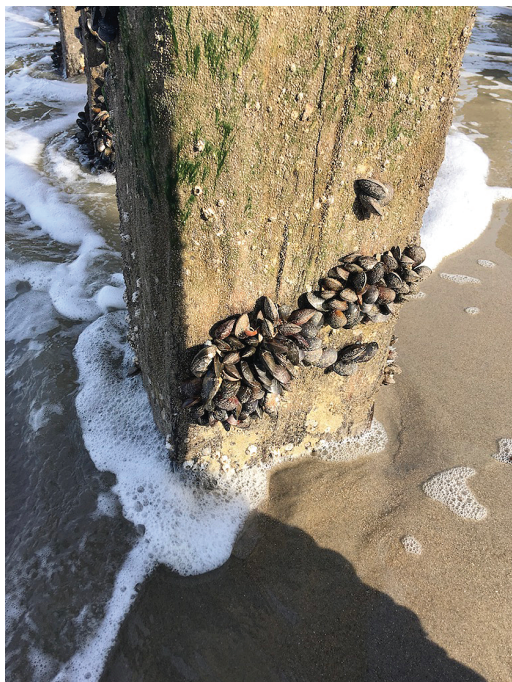
Figure 1.5 Mussels adhesive bonded to a wooden pile in the North Sea near Domburg, the Netherlands. Source: Dr. Jürgen Klingen, Aboso-Consulting.
