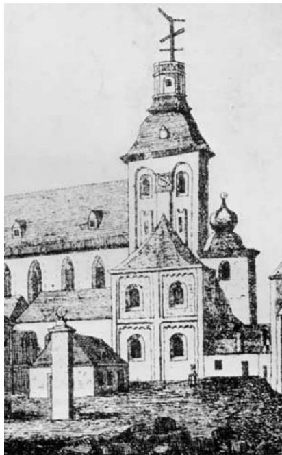
Fig. 1.10 Historic station No. 51 of the Berlin–Cologne–Coblenz optic-mechanical ‘sight’ transmission line on the tower of the St. Pantaleon church, Cologne. Picture by Weiger (1840).
