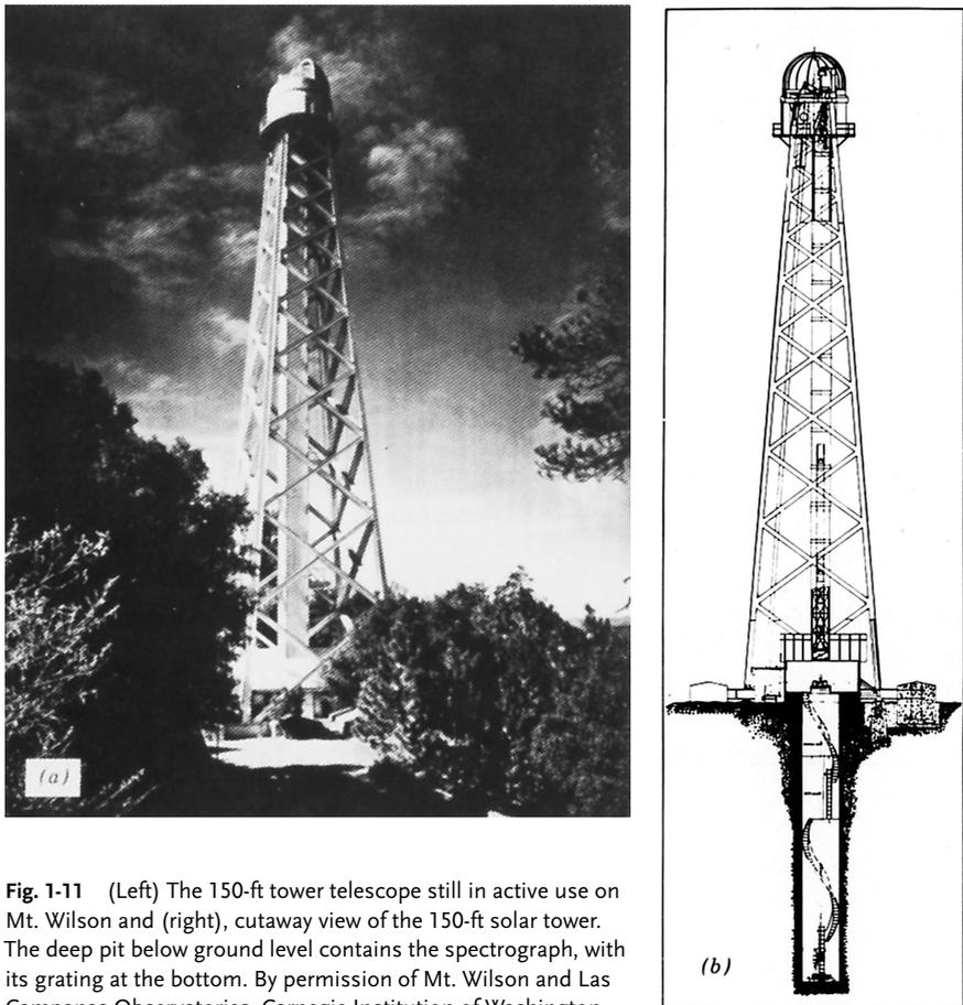
**Fig. 1-11** (Left) The 150-ft tower telescope still in active use on Mt. Wilson and (right), cutaway view of the 150-ft solar tower. The deep pit below ground level contains the spectrograph, with its grating at the bottom. By permission of Mt. Wilson and Las Campanas Observatories, Carnegie Institution of Washington.
