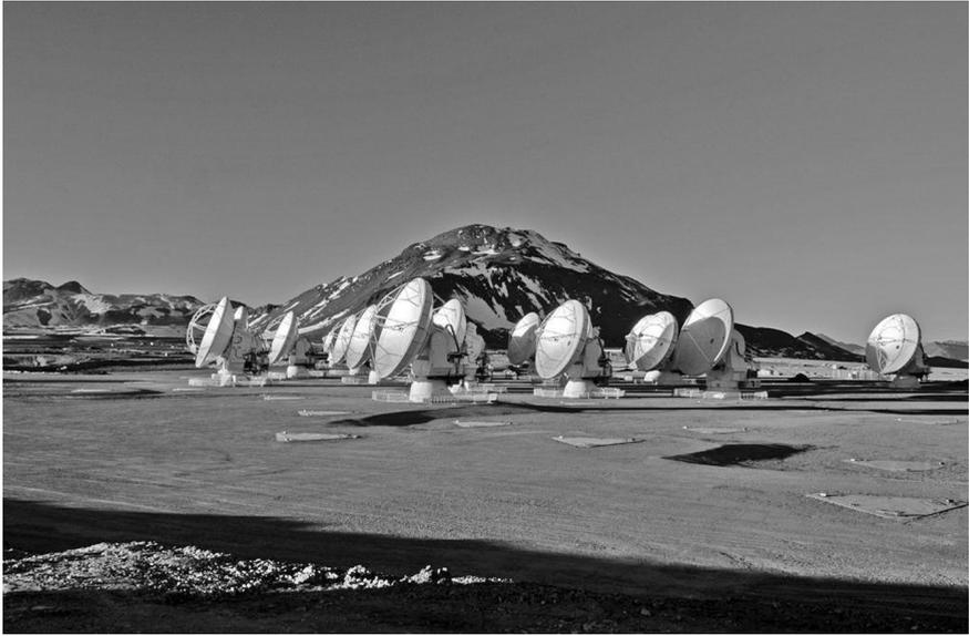
**Fig. 1-21** The Atacama Long Baseline Millimeter Array (ALMA) in its present form, with 39 of the 64 12-meter aperture dishes in place. The site in the Chilean desert is located at 5,000 meters altitude. By permission of the National Science Foundation
